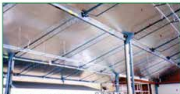
ROOKABURRA MANUFACTURING PLANT - REFURBISHMENT
